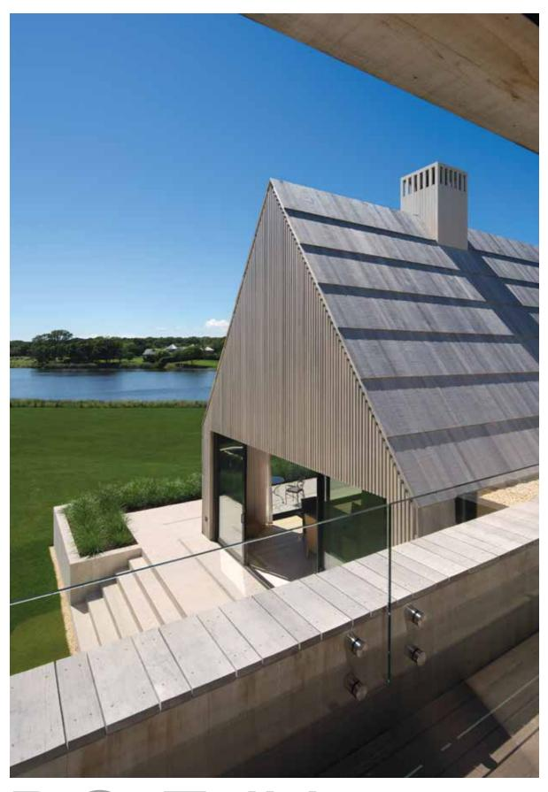
Plinth elevates structure above flood plane.
