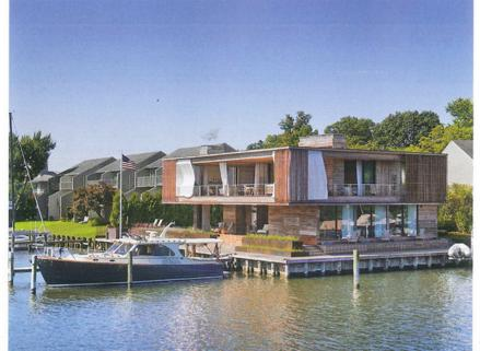
continuous stainless-steel track that runs all around the perimeter of the second floor. Then come panels of glass (or screen) that pocket into walls. Linen curtains and shades comprise the innermost layer. The owners can open the house completely, reveling in the view of the bay and letting the breeze blow through, or they can close themselves off, partially or fully.
